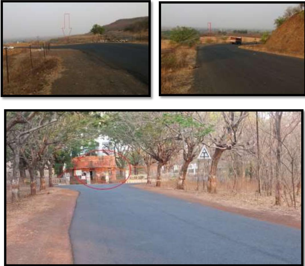
**Figure 10** Absence of Right/Left hand curve, chevron signs, Crash Barriers at a horizontal sharp curve
