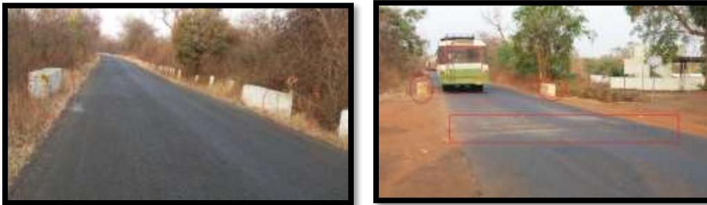
**Figure 6** Presence of speed breakers not indicated, fixed road side Hazards
