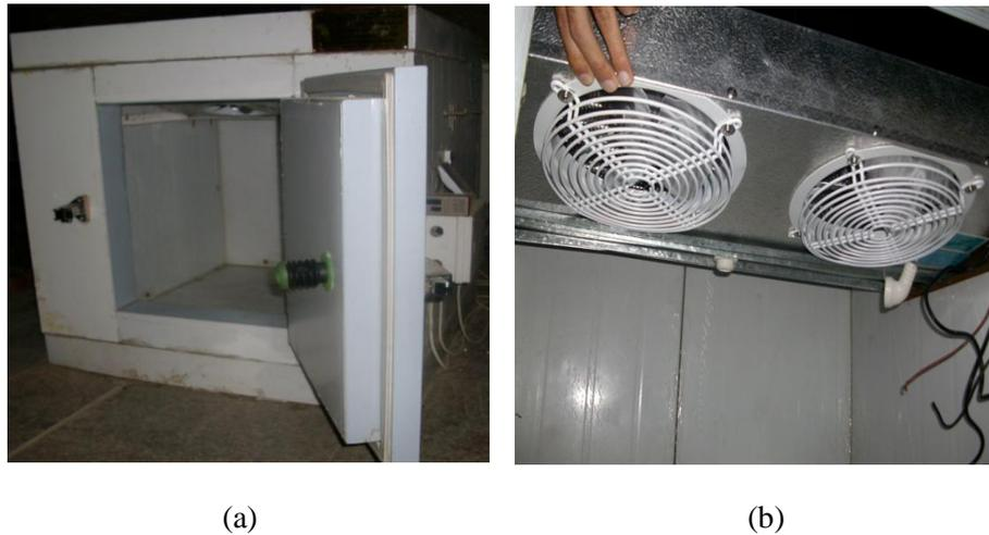
**Figure 1** (a) The cold storage and (b) The evaporator and fans (inside unit).
