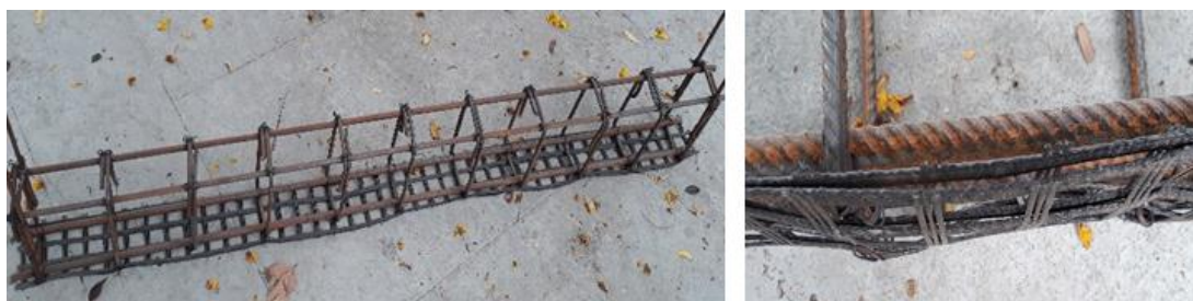
Figure 3 Geogrid layer as reinforcement
