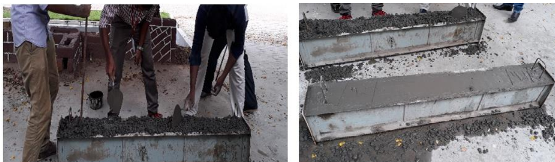
Figure 4 During and after casting of beams
