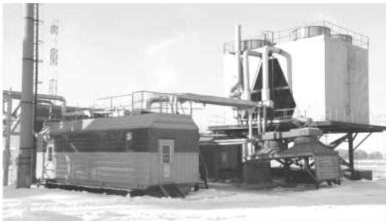
**Figure 1.** Heat recovery unit with a capacity of 500 kW at the Chaplygin compressor station LLC 'Gazprom transgaz Moscow'
