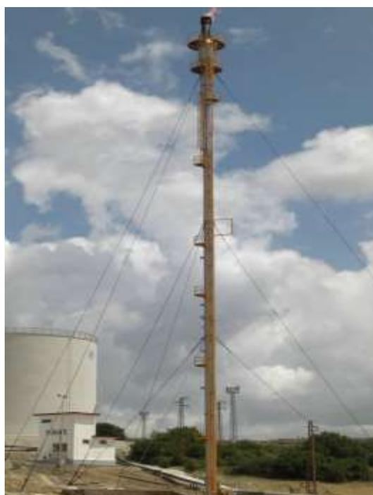
**Figure 1** General view of a typical flare stack supported using guy wires
