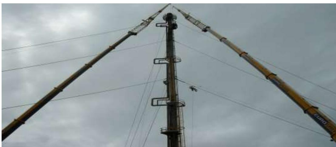
**Figure 2** Works on a flare stack using cranes and baskets, combined with rope access techniques for the inspection and lubrication of guy wires
