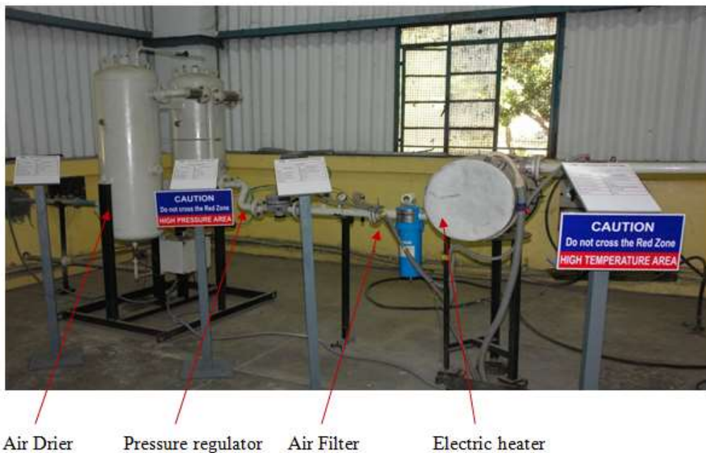
Figure 2 Components of ECS test rig
