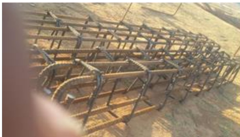
Figure 9 Reinforcement for beams
