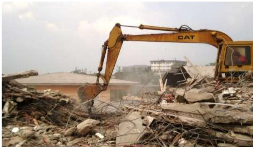
**Figure 1.** Collapse site of a 5-storey building due to excessive loading, Nkoldongo, Yaoundé (Tchamba and Bikoko, 2016)
