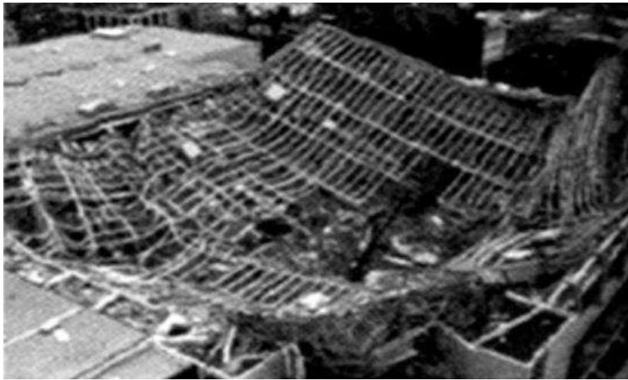
**Figure 3.** A view of the structure of the roof collapse due to design errors (Kobiela et al., 2015)
