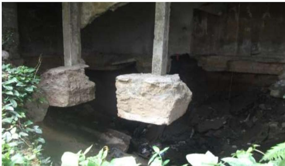
**Figure 2.** Foundation failure due to Erosion (Tchamba and Bikoko, 2016)
