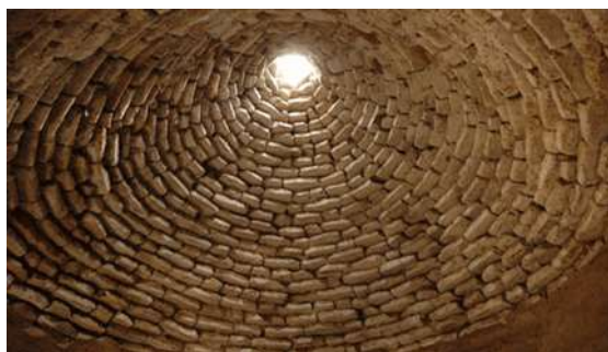
Figure 7 Top opening, source of natural lighting and helps the hot air flow to escape. [21]
