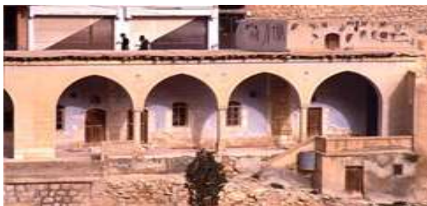
Figure 12 Loggia house from Syria. [20]
